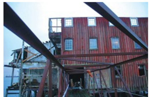
Before the storm, a boat hoist anchored the southwest corner at left. Fierce gusts as well as driving waves eventually led to its collapse.
